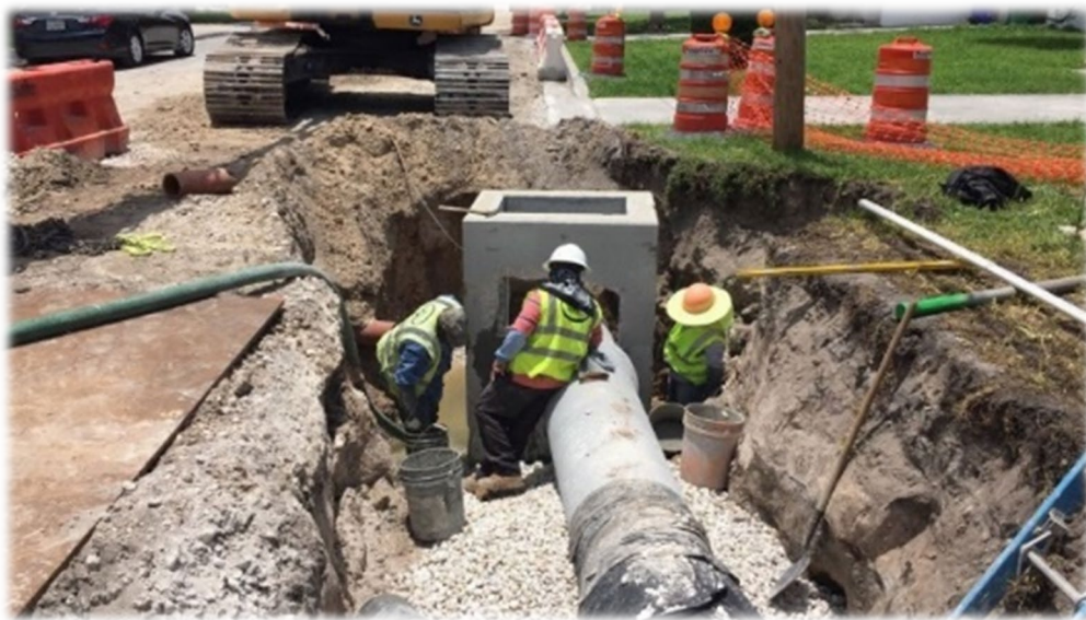
Drainage improvement project completed in Washington Park
