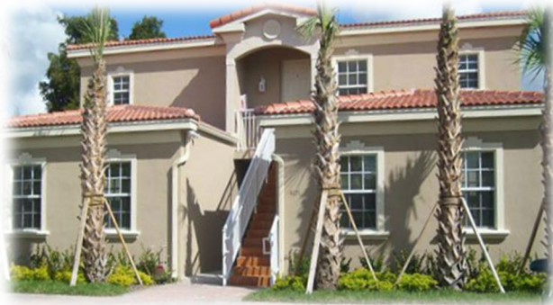
Woodside Gardens in Coral Springs An affordable housing development for young adults aging out the foster care system.
