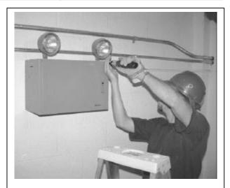
**Remove Panel Door Fasteners**
