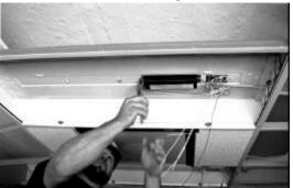
Cut wires and remove ballast.
