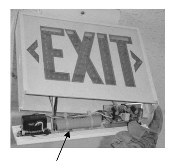
Nickel Cadmium Battery Pack in Exit Sign
