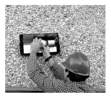
HID Bulb may be removed by unscrewing from fixture. *Note*: Outdoor lighting unit will need to be removed to remove ballast.
