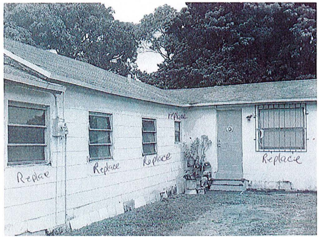
Replace 4 east side windows
