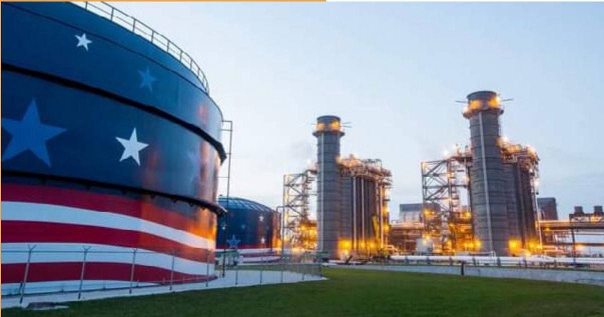
Port Everglades Next Generation Clean Energy Center, Fort Lauderdale, FL.
