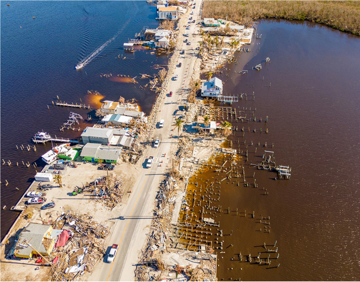
Aerial drone inspection photo of Pine Island Road, Matlacha, FL, showing Hurricane Ian aftermath damage and debris from flooding and storm surge. Photo Felix Mizioznikov / Dreamstime.com
