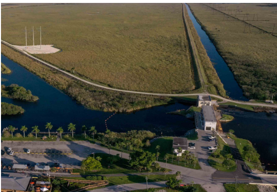
South Florida Water Management District pump station, Everglades Conservation Area 3 / South New River Canal. Photo: Paul Krashefski / Broward County Natural Resources Division
