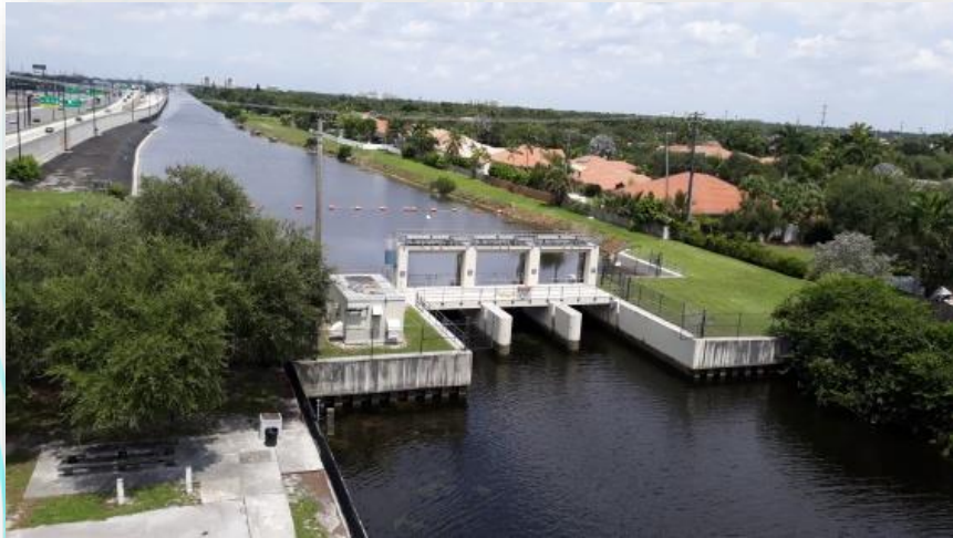
Gravity driven structure
