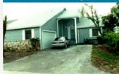
Level 2 - Major damage; habitable
