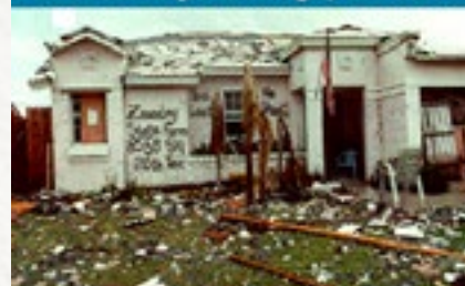
Level 3 - Major damage; uninhabitable
