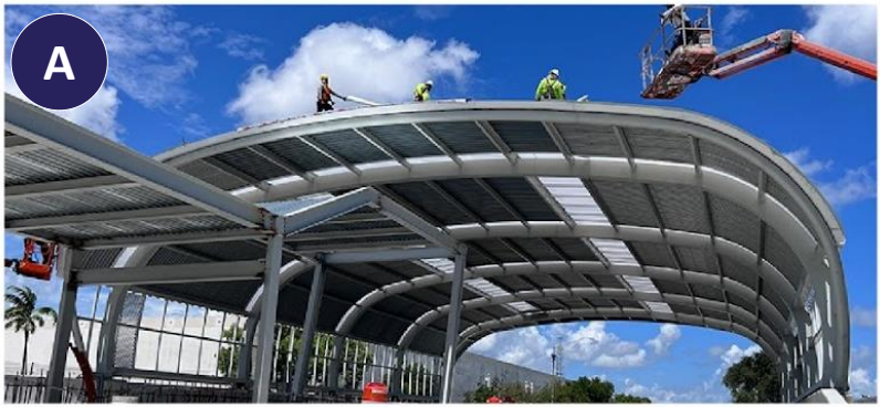
South Corridor: Bus Transit, under construction
