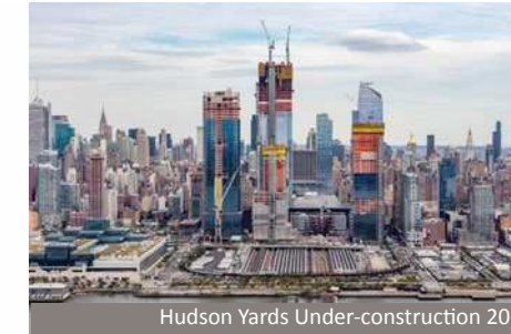
Hudson Yards Under-construction 2018
