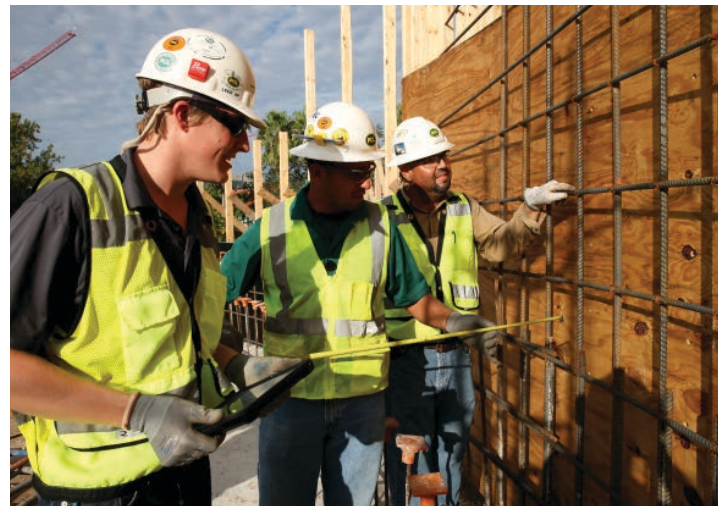
Civic Unity Partners Confirming Quality During Construction
