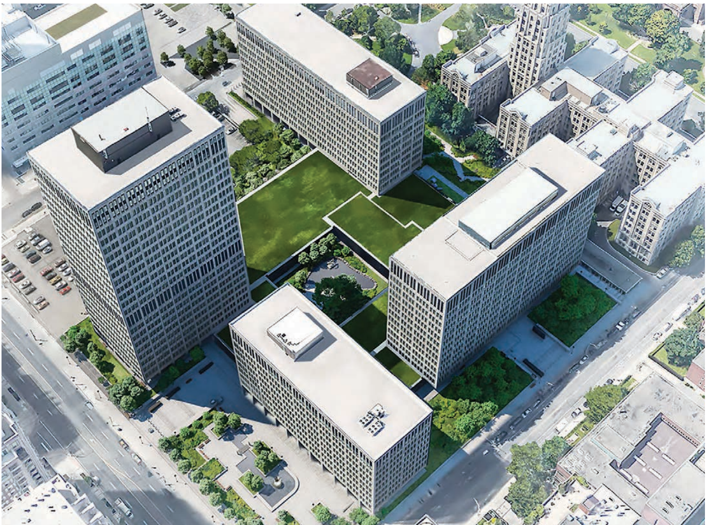
Figure 7: Macdonald Block Government Campus Renewal—DBFOM, Fengate, PCL Investments and PCL Construction
