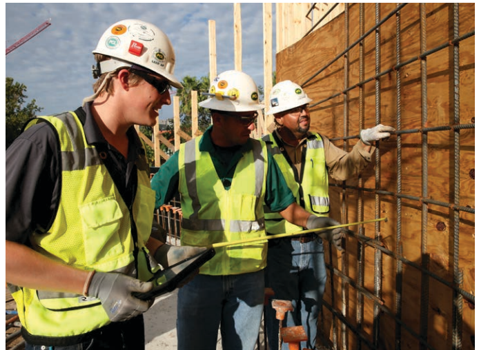
Civic Unity Partners Confirming Quality During Construction
