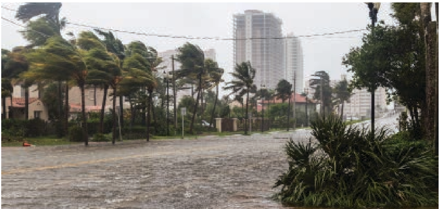
Impacts of flooding during a storm in Fort Lauderdale.
