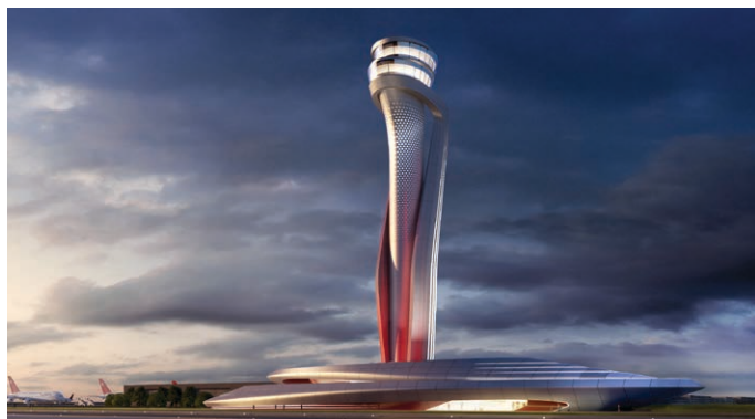
Istanbul Air Traffic Control Tower, AECOM & Pininfarina
