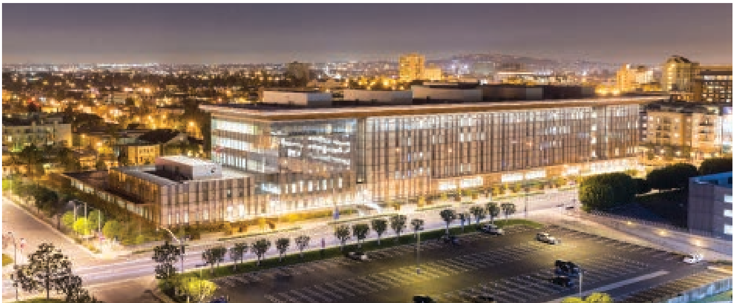
Award Winning George Deukmejian Federal Courthouse - Long Beach, CA
