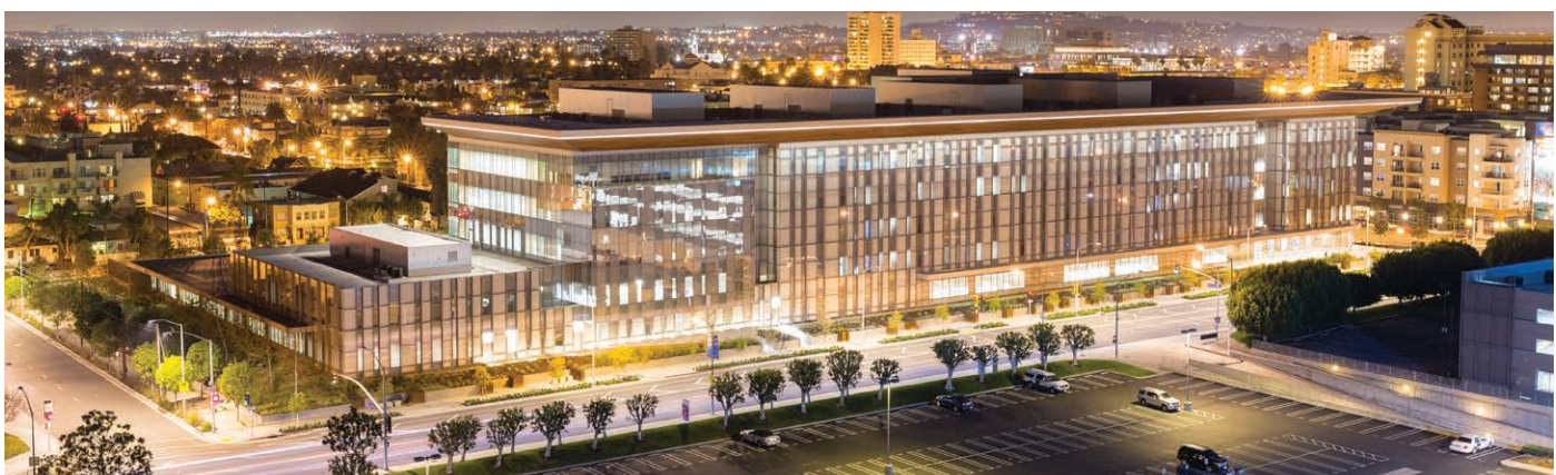
Award Winning George Deukmejian Federal Courthouse - Long Beach, CA
