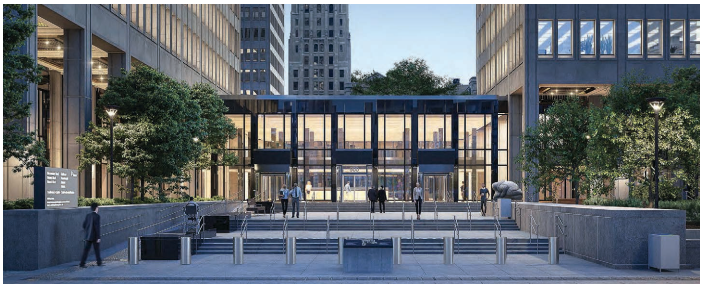
Figure 9: Macdonald Block Government Campus Renewal - Fengate, PCL Investments and PCL Construction
