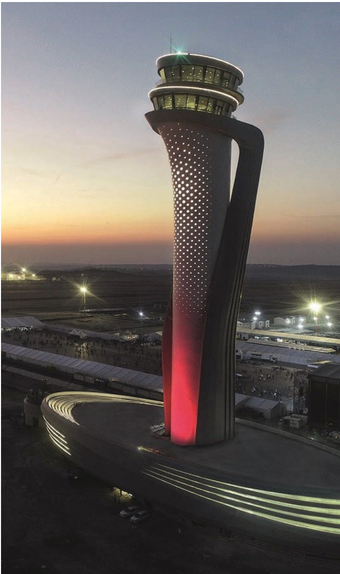
Istanbul ATC construction
