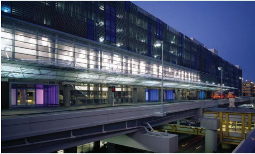
Consolidated Rental Car Facility - Fort Lauderdale, FL
