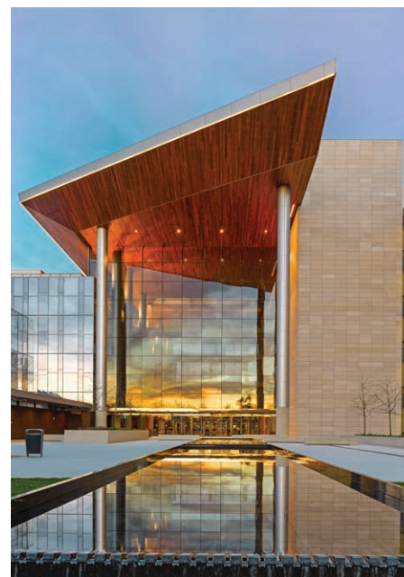
George Deukmejian Federal Courthouse
