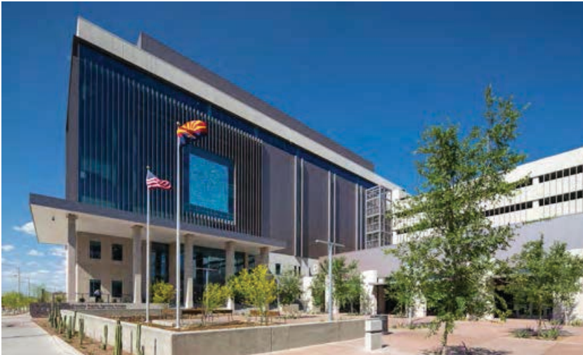
Joint Courts Complex for Pima County and City of Tucson, AZ
