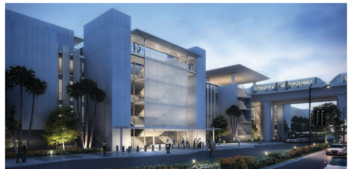
Figure 6: LAX Consolidated Rent-A-Car (ConRAC) — DBFM Fengate, PCL Investments and PCL Construction
