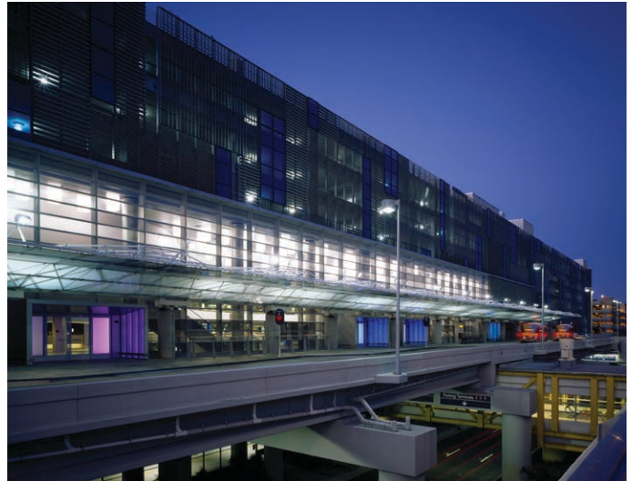
Consolidated Rental Car Facility - Fort Lauderdale, FL
