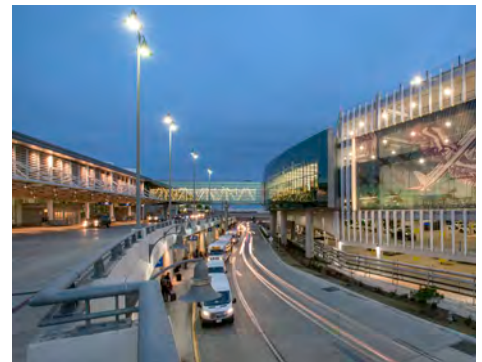
San Antonio International Airport ConRAC and Parking Garage, San Antonio, Texas
