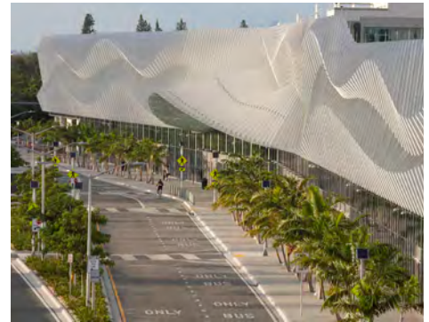
Miami Beach Convention Center - LEED Silver Miami Beach, Florida
