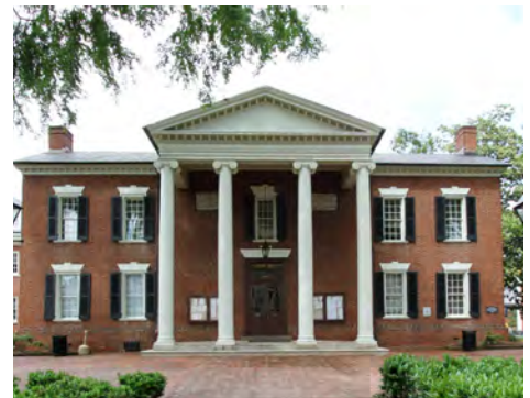
Albemarle County Courts Complex Addition and Renovation, Charlottesville, Virginia
