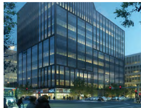
Richards Boulevard Office Complex Sacramento, California
