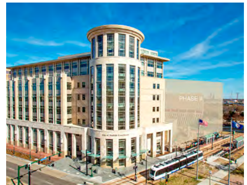
Norfolk Consolidated Courts Complex Norfolk, Virginia
