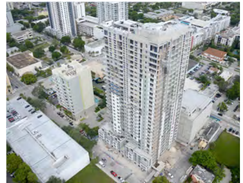
The Rise at Flagler Village Fort Lauderdale, Florida
