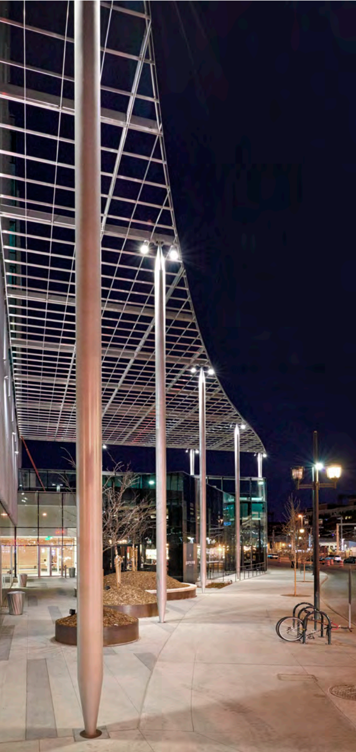
Photo: Union Tower West | Denver, CO
