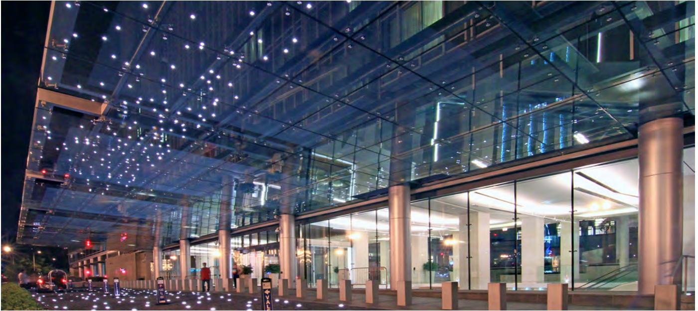
Marriott Marquis Washington, General Contractor, Hensel Phelps
