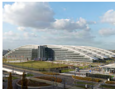
NATO Headquarters Brussels, Belgium
