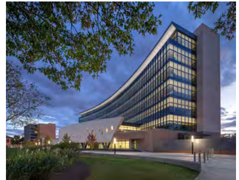
Johnson County Courthouse - WELL Principles Olathe, Kansas
