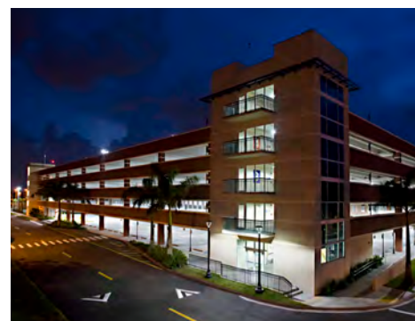
Broward College A. Hugh Davis Parking Structure, Davie, Florida
