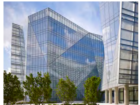
Benjamin P. Grogan and Jerry L. Dove Federal Building, Miramar, Florida
