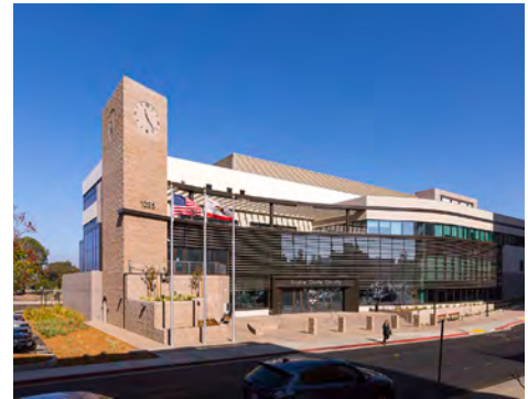
Contra Costa County Administration Building Martinez, California with Hensel Phelps
