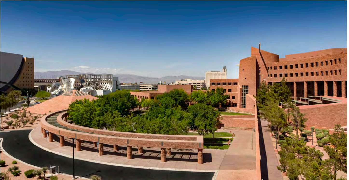
Completed Exterior of Amphitheater
