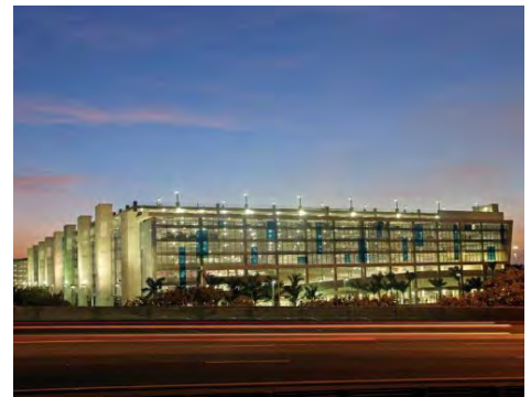
Cypress Parking Garage Fort Lauderdale, Florida
