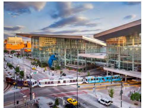
Colorado Convention Center Denver, Colorado
