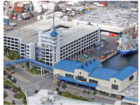
Port Everglades Parking Garage Connector Bridges
