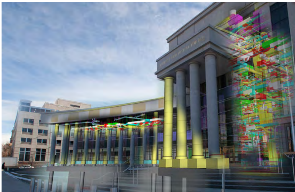
Ralph L. Carr Colorado Judicial Center, Denver, Colorado 2013 AIA TAP BIM Award - Delivery Process Innovation Outstanding Project Success Through Collaboration
