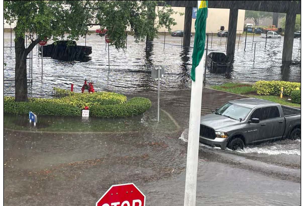
Flooded FLL Airport Perimeter Road on April 13, 2023
