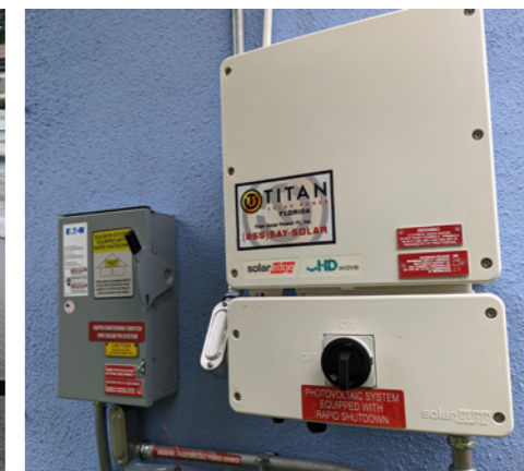
Solar roof panels and a wall-mounted SolarEdge HD Wave Inverter, converting direct current (DC) electricity from the solar panels to alternating current (AC) electricity for home use.
