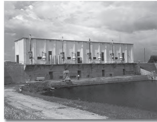
By 1960, six pumping stations are serving the dual purposes of flood control and water supply. Construction of the Central and Southern Florida Project creates the Everglades Agricultural Area (EAA) south of the lake and water conservation areas between the EAA and the east coast.
